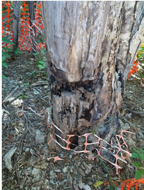
8: U041_Wood damaged by termite
